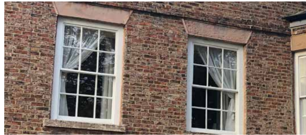
ORIGINAL SASH WINDOWS
